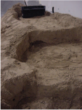
Sculpt dirt in stream area before installing liner
