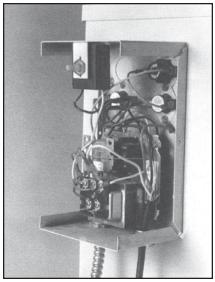
5a. Attaching furnace control center box. To separate outer cover, remove two (2) side screws and pull off black rheostat knob. Attach box to left side (facing feed door) with four (4) self-threading screws. One screw in each corner. (NOTE: Furnace control center is designed for left side attachment. Should space prohibit such, reversing shrouds for right side installation is possible, however, control wires from box will have to be 5b. extended.)
