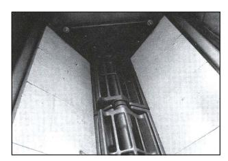
12. **Installing Firebrick:** Place 5 bricks on each side (10 brick total). The bricks tuck under firebox seem.
