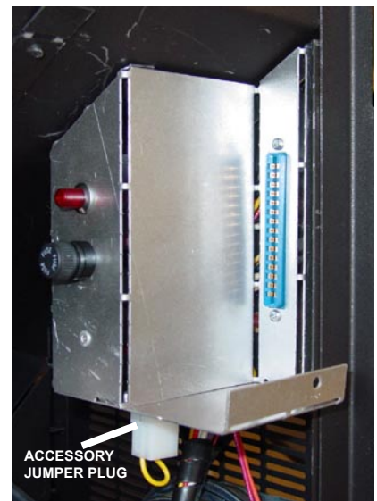
ACCESSORY JUMPER PLUG ON THE JUNCTION BOX.
