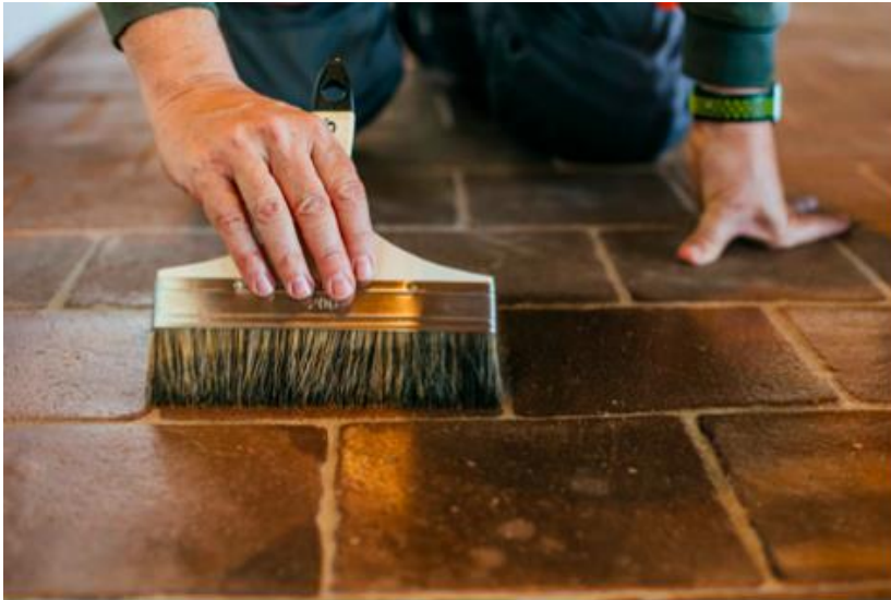
Final finish of the cleaning process and protection of the floor.
