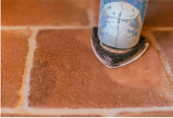
1.6. Detail of terracotta floor in the process of being cleaned.
