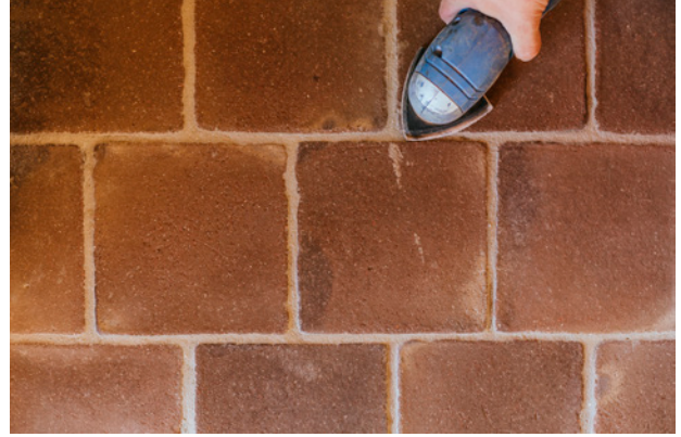
1.6. We will use the punch or sander to remove stains that have not been removed in the cleaning.
