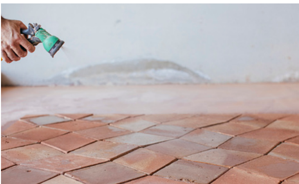
Wetting of pieces prior to grouting
