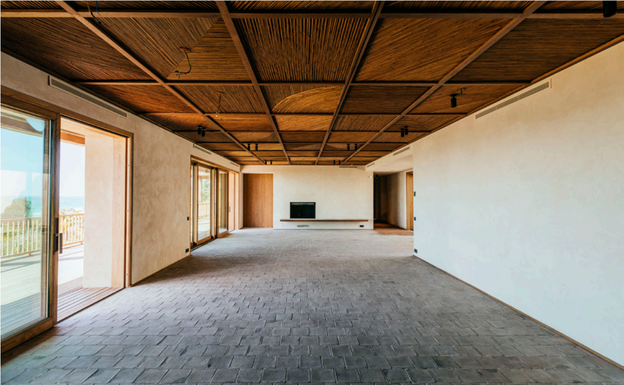
Before cleaning and protecting
