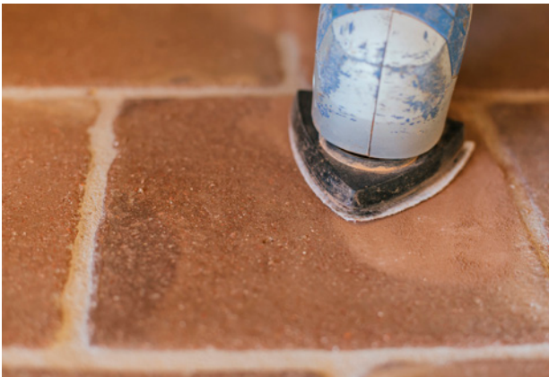
1.7. Detail of stain removal with the sander.
