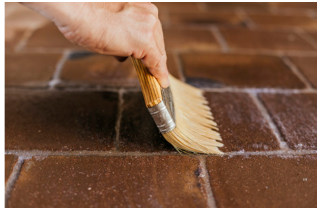
2.2. Applying the product manually.
