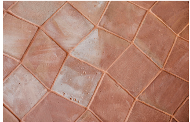
Preview of final cleaning
