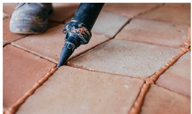
Joint sealing with grouting material
