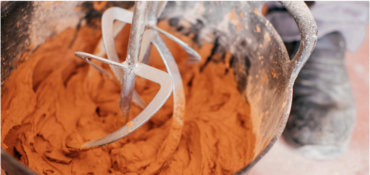
Adhesive mixing operation
