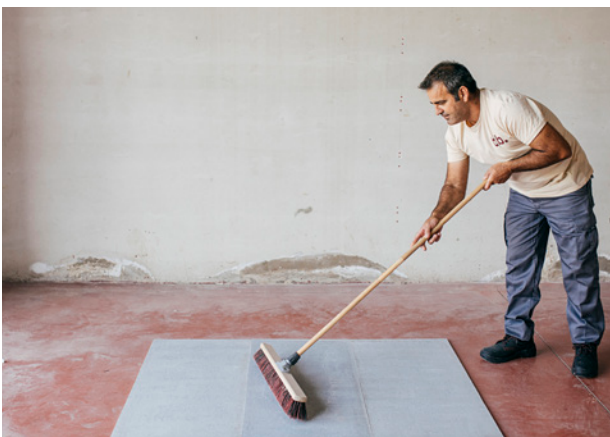
Laying support cleaning
