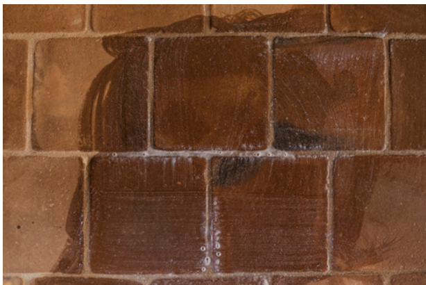
2.3. Application detail of the protective product.
