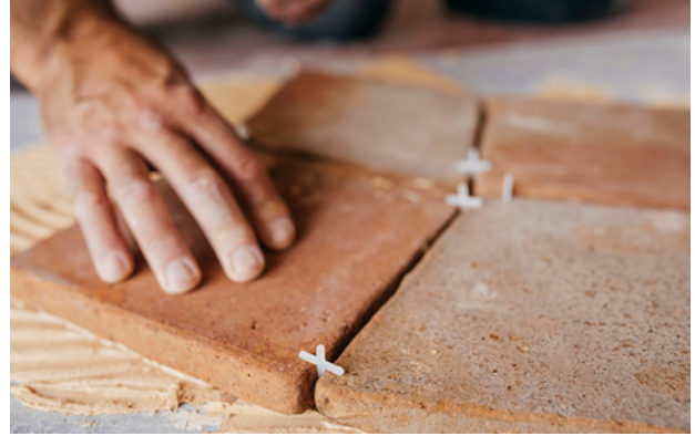
Tightening of tile joints
