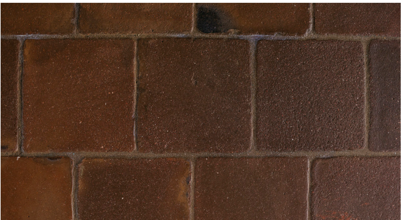
Final finish of the cleaning process and protection of the floor.
