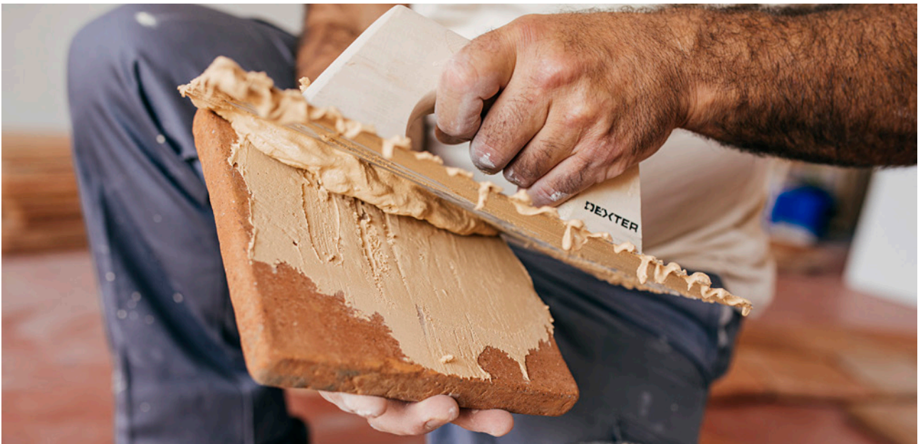
Adhesive Application in the back of the tile
