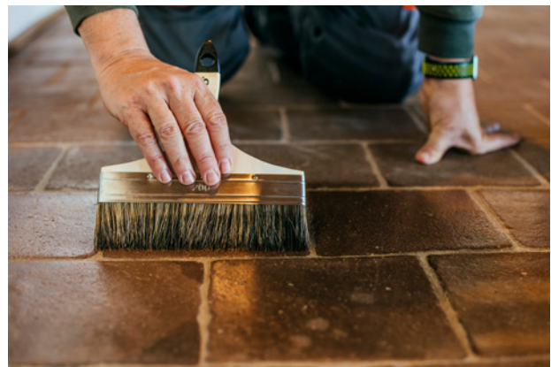
3.2. Application of the product generating a thin and diluted layer.
