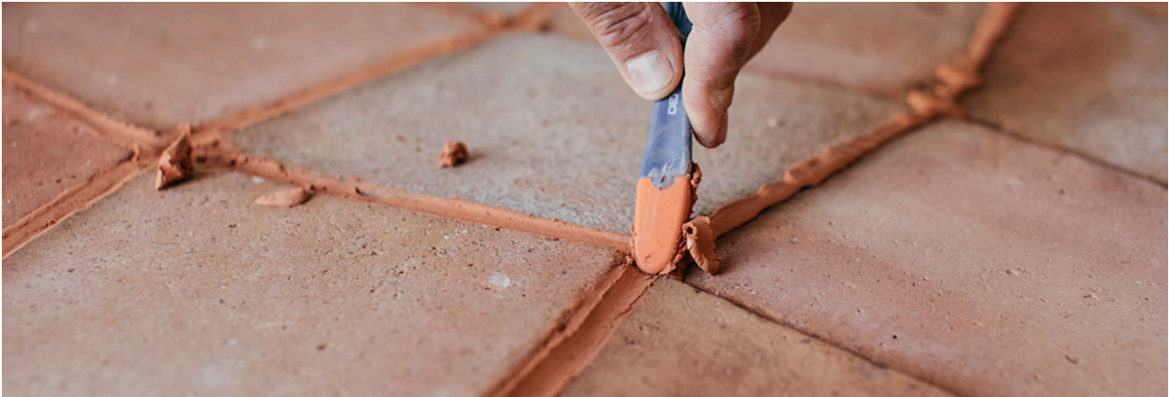
Llaguero for removal of excess grouting material
