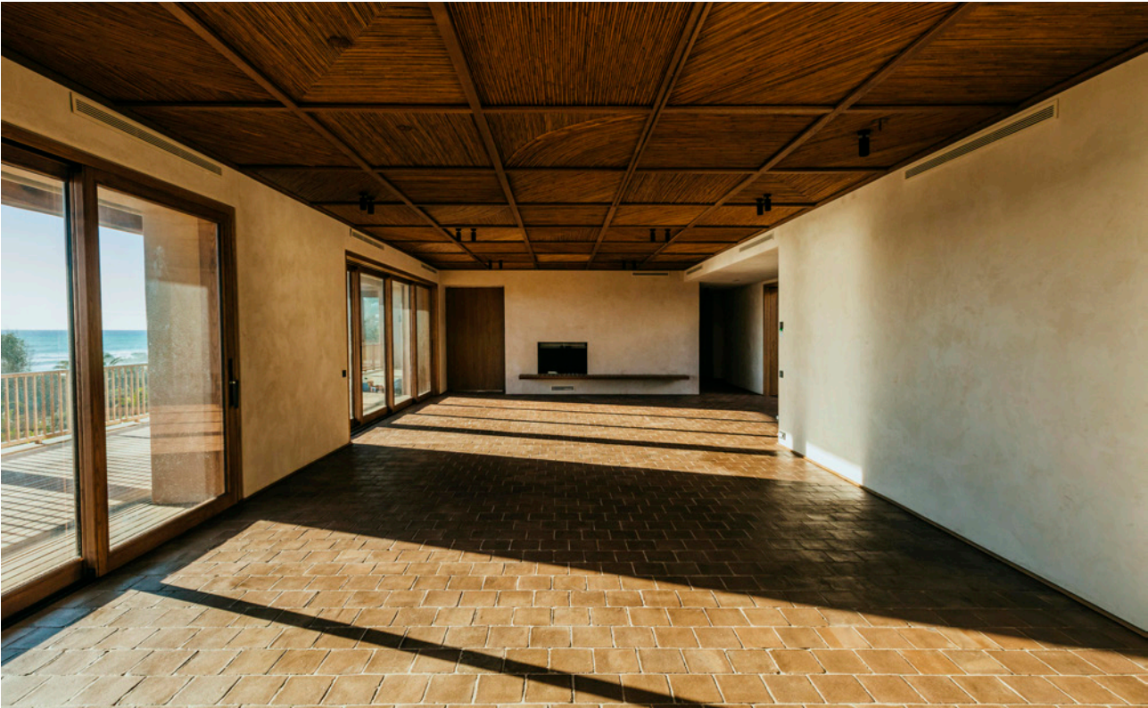
After cleaning and protecting
