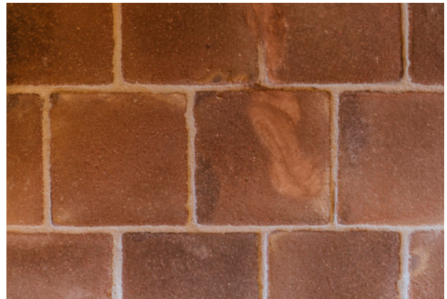
1.8. Detail of terracotta floor in the process of being cleaned.
