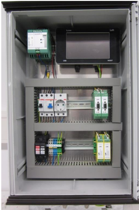
Example of a standard Lufft UMB cabinet as well as examples of the grounding of the shield
