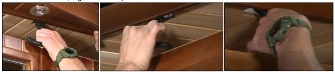
Once all the cables have been threaded through the Roof Cap holes, place the Roof Cap securely onto the walls of the sauna.
