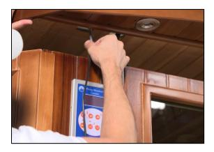
Feed the remaining black heater plugs through the pre-drilled holes on the Roof Cap located on the right side of the Middle Front Wall, Right Back Wall, and Left Back Wall.
