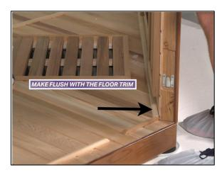
The Middle Front Wall includes three metal guides on each side to accommodate the addition of the Left and Right Front Walls.
