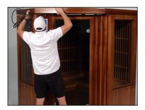
On the left-hand side of the Middle Front Wall, above the Control Panel are six cables. Feed all six cables through the hole in the Roof Cap.
