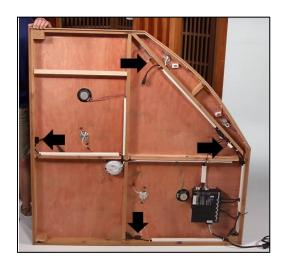
Carefully place the Roof Cap on the top of the sauna. It does not need to sit flush with the walls at this time since the power cables need to be fed through the predrilled holes.
