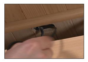
Do the same with the five remaining black heater plugs located one on each side wall and two on the Back Wall.
