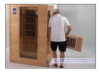
A label is located on the top of the Bench Heater Panel indicating which side needs to be placed facing up.
