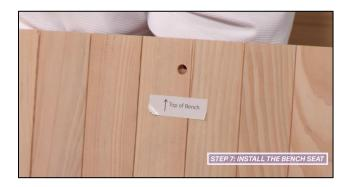
Bring the Bench Seat in through the right side of the sauna, then lay horizontal for installation. Wait to install the anchoring screw into the bench seat until later.
