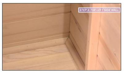
The Left Side Wall includes trim pieces on both sides that will wrap around the Back and Front Walls.
