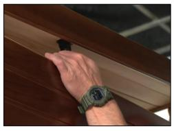
Once all the cables have been threaded through the Roof Cap holes, place the Roof Cap securely onto the walls of the sauna.
