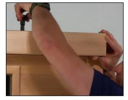
Once all the cables have been threaded through the Roof Cap holes, place the Roof Cap securely onto the walls of the sauna.
