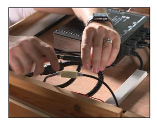
Continue to make the additional power cord connections around the top of the sauna.
