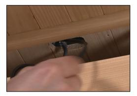
Feed the remaining black heater plugs through the pre-drilled holes on the Roof Cap located on the right front, Right Side Wall towards the back of the wall, the middle back of the Roof Cap and the Left Side Wall towards the back of the wall.
