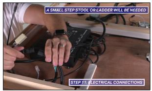
Continue to make the additional power cord connections around the top of the sauna.
