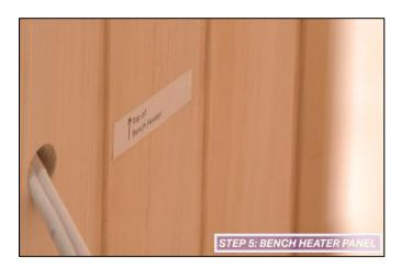
Place the Bench Heater Panel between the guides found on each side of the bottom of the Floor Base with the heater panel facing the door. Lastly, ensure the heater cord is placed behind the Bench Heater Panel.
