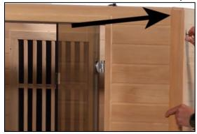
Insert the remaining installation bolts into the predrilled holes to connect the Right Side Wall with the Front and Back Walls. Again, only finger tighten the bolts. If needed, use a screwdriver to tighten the bolts but do not tighten completely.
