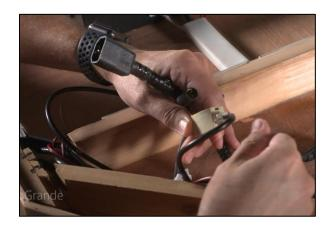
Continue to make the additional power cord connections around the top of the sauna.
