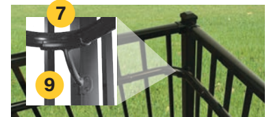
Inside Corner Mount & 90° Elbow Detail
