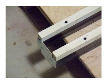
Larger holes in Studs face outward towards drywall. Center the rear studs in opening between Front Studs and Rough Opening.
