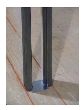
5. Check Door Fit before Installing Drywall. Make necessary adjustments to upright studs if needed. Apply desired drywall. Drywall should be flush with edge of opening. Use provided special self-tapping screws to attach Drywall to studs. If using your own screws, they can not be long enough to protrude into pocket, or Doors will be Damaged. (Screws Provided #8 x 1 1/4")
