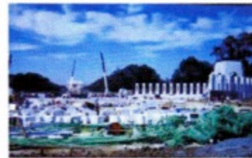
Construction Progress (Sep. 25, 2003)
