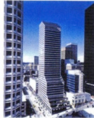
Key Tower Building
