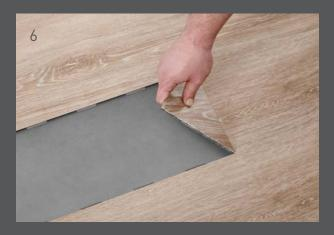
Pry the first plank section loose by inserting a putty knife in the cut running down the center of the plank. Gently unclick the first plank section from the adjoining planks;
