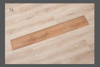
Place a heavy weight on the newly inserted plank and allow to cure undisturbed for 24 hours;
