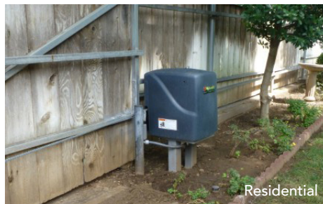
SlideSmart DC 15 SlideSmart DCS 15F (solar) 1,500 lb (680 kg) gates 0.75, 1 or 1.25 ft/s (23, 30 or 38 cm/s)
