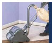
TIP: If starting with a 24 or 40 grit belt, never skip a grade in the sanding process, you must use all grits available before finishing with a 120 grit belt.
