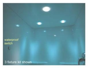
The steam room lighting kit is designed to allow up to a total of 7 light fixtures connected, in a daisy chain configuration with approx. 6 feet of wire between each fixture. Low voltage light fixtures easily connect together with pre-installed locking connector terminals. Control Switch is waterproof and is recommended to be installed near steam room entrance door. Use appropriate hole saw type and size for drilling through steam room ceiling material.
