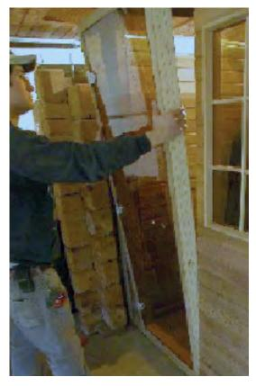
(1) Bottom sill plate should be of treated wood. Where sill plate meets floor must be caulked well to prevent water leakage in the case of excessive water use.
