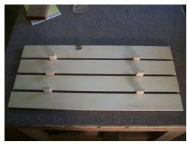
Step 2) Use a framing square to align the the end of the valance and determine how many lateral support pieces  $(1" \times 2")$ you will need. Figure at least one every 30".
