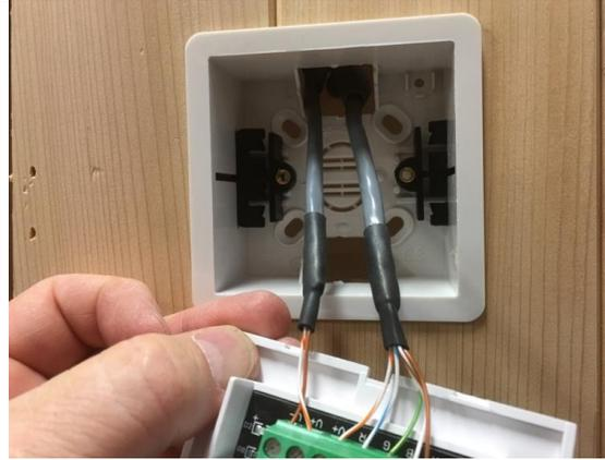
Insert the two CAT5 cable ends into the upper or lower opening in your enclosure. (upper will allow more cable to be in the wall)
