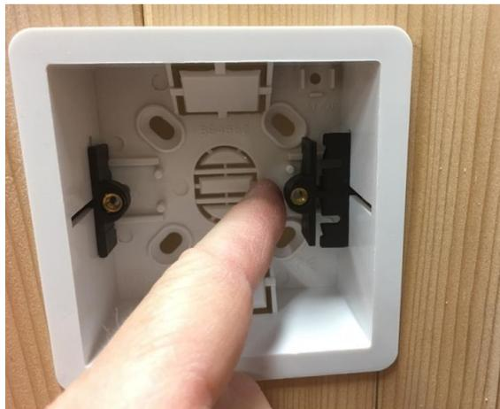
When satisfied with the fit of the enclosure in the sauna wall, push the two black tabs outward and pull each forward until they make contact with the back of the wall surface.
