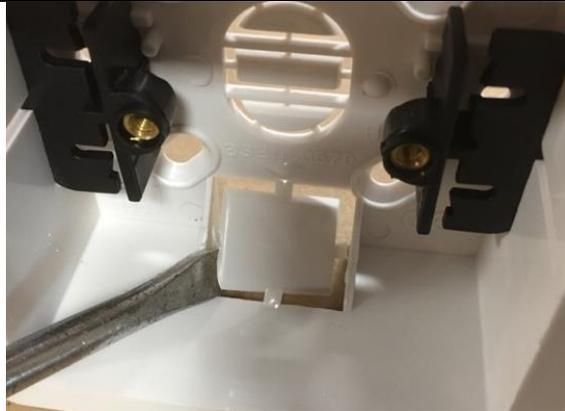
Using a screw driver or utility knife, carefully remove the upper and lower knock-out tabs so the control cables can be routed outside of the enclosure.
