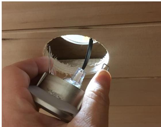
Using a drill-mounted hole saw, cut a 2 3/4" hole at each of the desired locations in your ceiling. Carefully compress the two spring clips on the fixture and insert them into the hole until they are past the thickness of the ceiling material. Slowly allow the clips to pull the fixture up into the hole to secure it to the ceiling.
