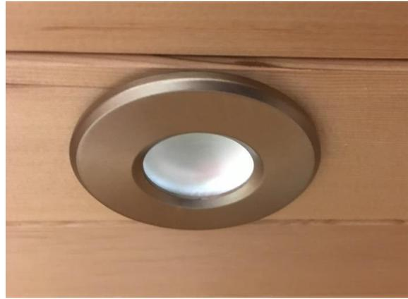
The silicone gasket should lie flat between the fixture and the ceiling. If it does not, pull the fixture down to remove any wrinkles in the fixture and re-install using the step described above.
