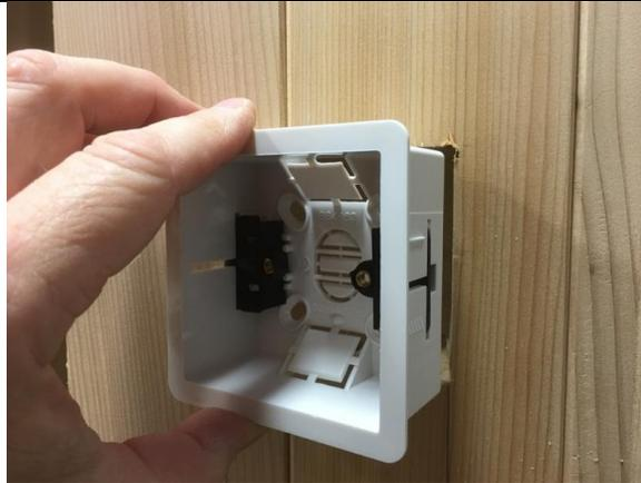
With wall material removed, pre-fit the flush mount enclosure to make sure it fits snug and level in the opening.
