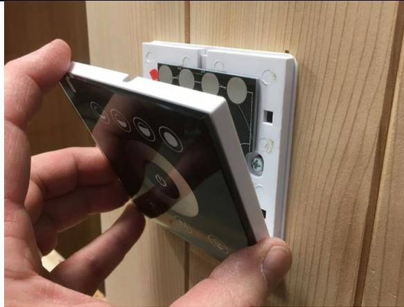
Snap the glass panel onto the control by aligning the notches on the bottom of the panel first then pivoting the glass panel horizontal. Use light pressure to “snap” the glass cover in place.
