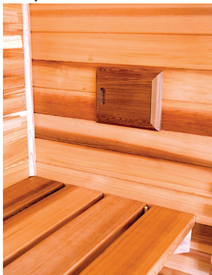
Inside view of installed Sauna Vent Kit. Outlet Vent is typically installed on Opposite wall about 1/3 up from the floor.
