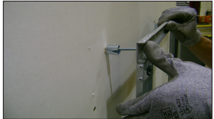
Figure 4.10 Installing Anchors in Hollow Wall
