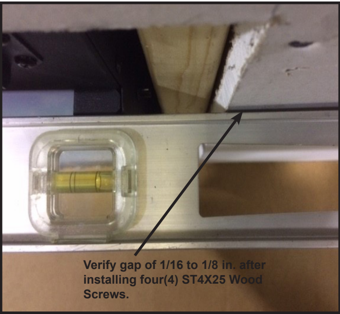
Figure 4.5 Adjust Bracket Location
