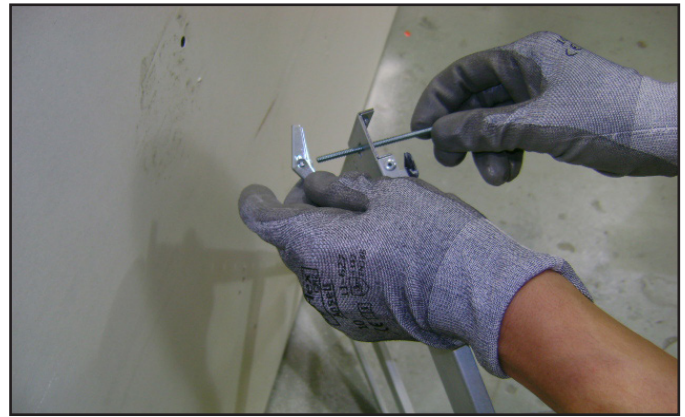
Figure 4.9 Toggle Bolt Installation through Mounting Bracket
