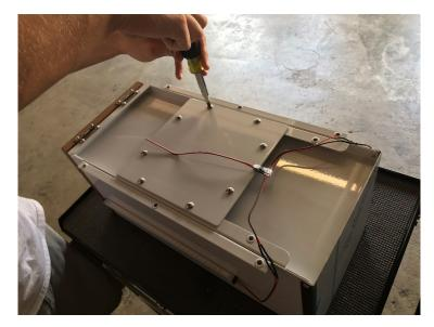
9. Once removed, a 1/4"- 3/8" diameter hole should be drilled into the center of the mounting plate. This is an aluminum plate, so drilling is rather easy with most standard drill bits. Take it slow to ensure safety.
