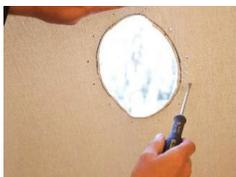
**STEP 5** - using a screwdriver, make a hole large enough for each of the screws to go through.
