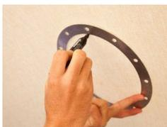
**STEP 3** - With a pen, draw around the INSIDE of the metal ring and mark where each of the holes is.
