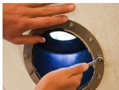
**STEP 6** - Screw on the flashing kit with one metal plate on each side of the tent. It can be left in place forever once installed.
