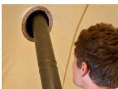
**STEP 7** - Push the flue through the flashing kit and connect it to the stove, making sure everything's straight.
