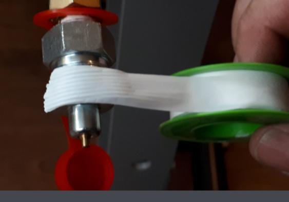
Now is the time to get some plumbers tape and use it on ALL connections you have to make in this guide. Be sure to wrap the tape in the same direction on the threads as you screw it in.
