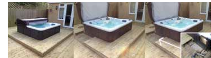
Ensure part of your decking can be removed in order to gain access for future repair or servicing
