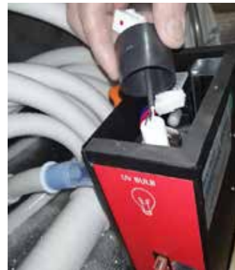
Step 4: Take out this black protective sleeve
