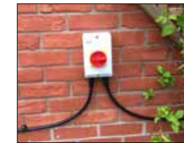
Rotary Isolation Switch (pictured). Make sure you have a qualified electrician prepare the electrics. Allow 5 metre slack to connect to Spa.
