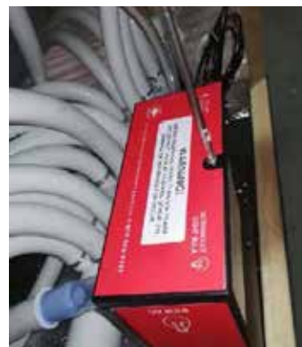
Step 8: Cover the red lid and install these 2 screws
