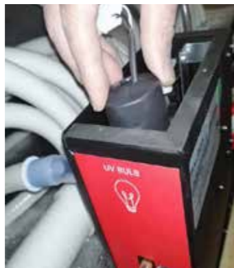
Step 6: Put the bulb inside the metal tube and cover it with black protective sleeve
