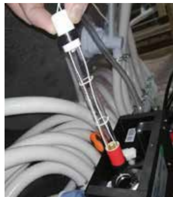
Step 5: Pull out the bulb to change it
