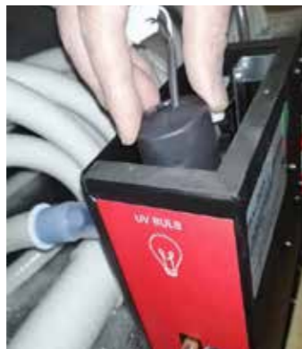
Step 6: Put the bulb inside the metal tube and cover it with black protective sleeve
