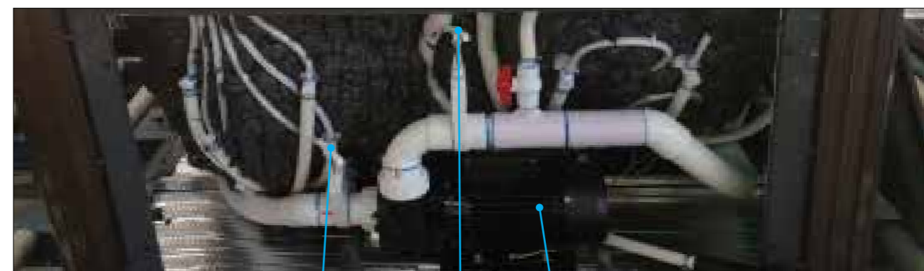
Slice valve Slice valve Pump
