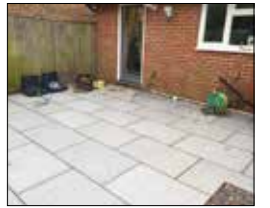
Ensure you have prepared a level concrete base or a properly fitted existing patio or decking with access to a drain.
