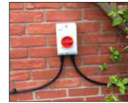
Rotary Isolation Switch (pictured). Make sure you have a qualified electrician prepare the electrics. Allow 5 metre slack to connect to Spa.
