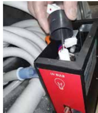
Step 4: Take out this black protective sleeve
