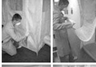
To open main entry doors, unzip side zippers to desired height. Roll door up; use Velcro® strips located above door to hold the roll securely. Be sure to close door immediately after passing through, and prior to opening the opposite door panel to prevent cross contamination.
