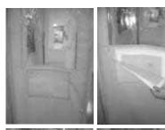
Close all openings and doors on unit. Turn on air handling equipment to create negative pressure in unit. If pressure created in unit is too great, open panel on side door to relieve pressure. Screen can then also be opened to pass objects through.
