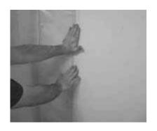
Step out of unit. Use tape or adhesive to hold flanges against wall. Flanges are located on both sides and top end of unit.
