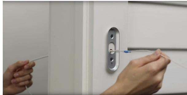
**Important:** Don't plug in the adapter yet. You might damage it if the wire ends touch each other. Keep it unplugged until you finish installation.
