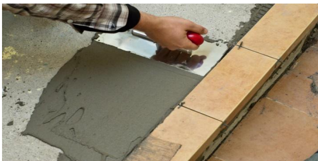
Apply Adhesive using Plain Side of Trowel
