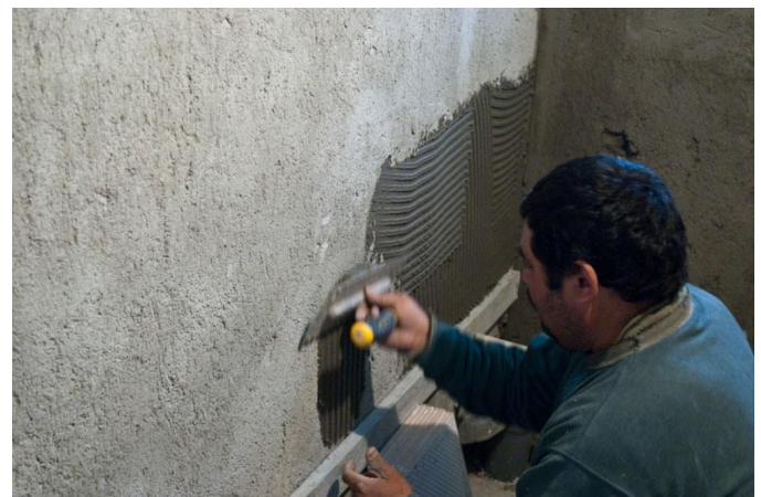
Application of BS Tileasy on Wall over smooth levelled / plastered surface.
