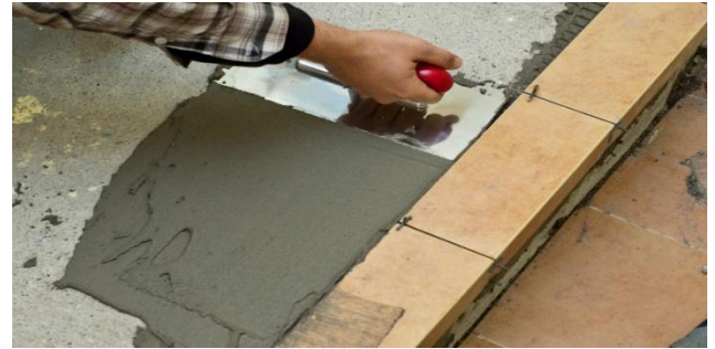
Apply Adhesive using Plain Side of Trowel
