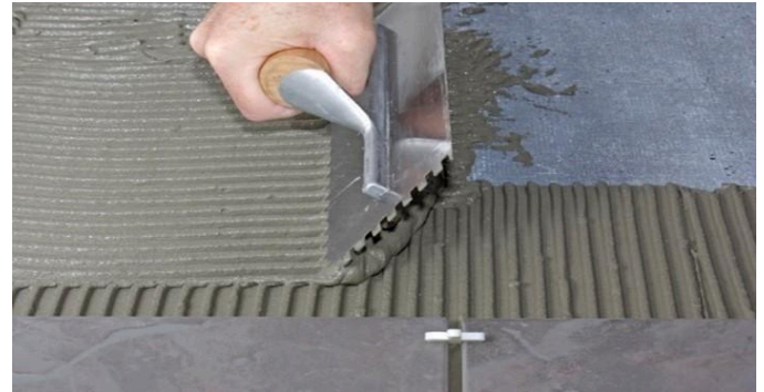
Use the Notch sized to control adhesive application as needed.
