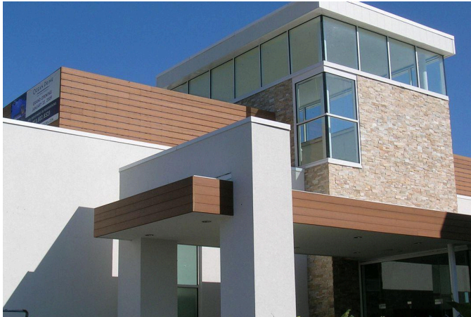
BS Tileasy HS used for Stone tiles application on Facade Wall.
