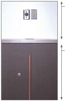
The receptacle, water shut-off valve and drain pipe must be within 3 feet (36") of the center of the location (footprint) of the machine.
