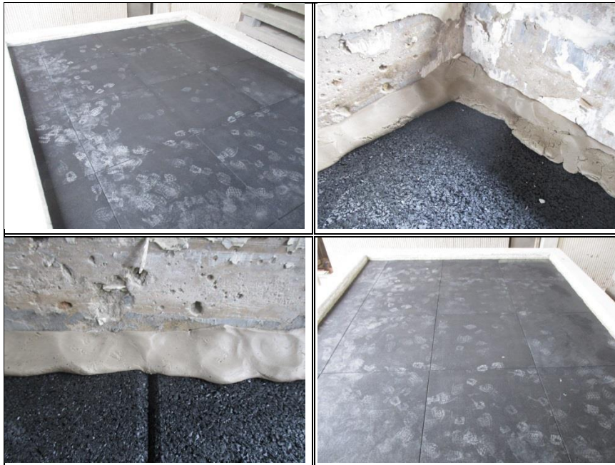
Images 5 to 12 Installation and sealing of the floor covering on the reference floor
