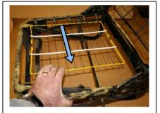
HOOK THE NEW WIRE FRAME ONTO THE SPRINGS ALONG ONE SIDE & SUPPORT IT WITH ONE HAND KEEPING IT TENSIONED SO THAT THE SPRINGS REMAIN ENGAGED.
