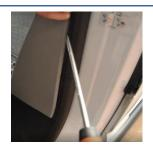
Next carefully release the panel using a flat head screwdriver – start at the bottom and work your way up.
