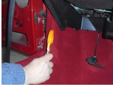
Glue the carpet to the scuttle and fit the bolts. You can use the blunt edge of an object to make sure the carpet sits in all of the groves.
