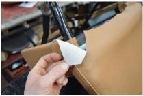
9) Now we look at the rear of the cover. Find the point where the rear frame cross member meets the rear leg. Place scissors into this corner & cut at approx.. 45°.
