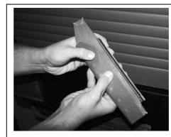
2: Before fitting the fillets (it doesn't matter which you fit first) bend the flaps over firmly to stretch them into the shape they will have to hold in the door.
