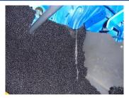
With the loop pile carpet, place the scuttle panel in place and mark where you need to trim. We would advise trimming in stages so not to cut off too much.
