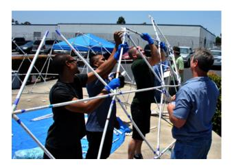
Step by Step <u>Instructions</u> to build a 5V Geodesic Dome Using Sonostar *hardcore* Geohubs. Builders can choose to either use the included stainless steel nuts and bolts to attach the hubs, or use PVC welding glue (for a permanent dome), or both.
