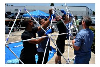
Step by Step <u>Instructions</u> to build a 5V 3/8 Geodesic Dome Using Sonostar **Mega** hubs. Builders can choose to either use the included stainless steel nuts and bolts to attach the hubs, or use PVC welding glue (for a permanent dome), or both.
