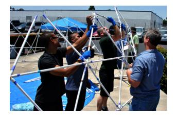
Step by Step <u>Instructions</u> to build a 5V 58 Geodesic Dome Using Sonostar **Mega** hubs. Builders can choose to either use the included stainless steel nuts and bolts to attach the hubs, or use PVC welding glue (for a permanent dome), or both.
