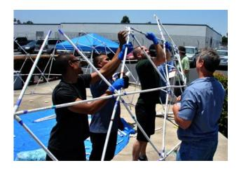
Step by Step <u>Instructions</u> to build a 4V Geodesic Dome Using Sonostar *hardcore* Geohubs. Builders can choose to either use the included stainless steel nuts and bolts to attach the hubs, or use PVC welding glue (for a permanent dome), or both.
