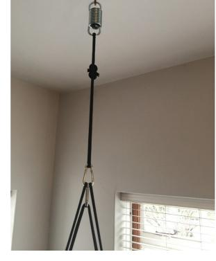
Example of SLING chair hanging mechanisms - in a concrete roof.
