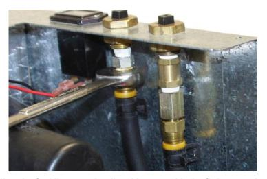
1. Align the fuel lines on the diesel burner with the fittings on the Hydro-Hot, and using a 11/16 inch wrench, tighten down both the supply and return fuel fittings.
