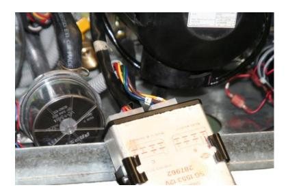
1. Locate the Diesel-Burner's Controller and disconnect both plugs. Failure to do so may result in the Diesel burner igniting.
