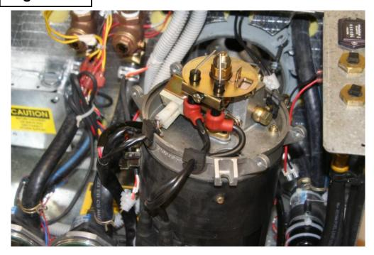
2. Carefully pull the Diesel-Burner away from the Hydro-Hot 4 to 5 inches before rotating the burner, and then remove.
