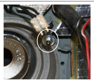
1. The Diesel-Burner is secured to the Hydro-Hot with two eye-bolt nuts that can be swung into place, after the diesel burner has been properly aligned and set in place.
