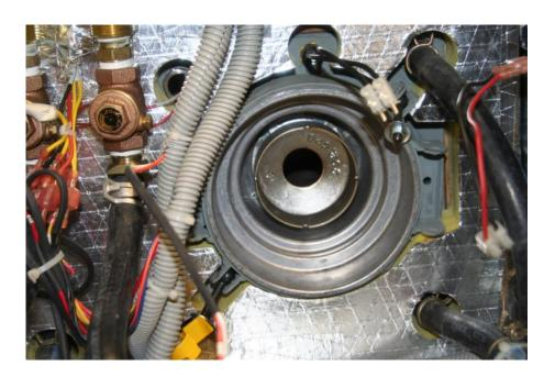
1. Reinstall the Combustion Chamber into the Hydro-Hot. Be sure to install the combustion chamber Seam in the 12:00 position. Failure to do so, may cause a crack to appear along the seam.
