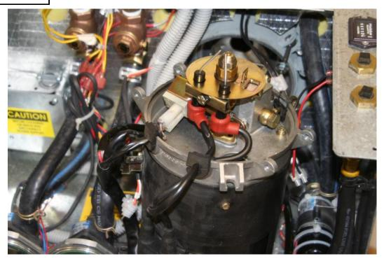
4. Carefully pull the Diesel-Burner away from the Hydro-Hot 4 to 5 inches before rotating the burner, and then remove.
