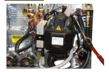
3. The Diesel-Burner is secured to the Hydro-Hot with two 10mm nuts that can be loosened, and swung out of the way by using a 10mm socket wrench with a 10 inch long extension.
