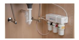
Turn the cold water on. Check for leaks and proper installation: place a towel under the filter unit and check for leaks. Allow water to run for 10 minutes to flush carbon fines.
