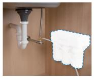
Unit Installation: Select a space under your sink for the filter unit that is at least 30cm from the bottom of your cabinet and allows for easy access to your cold water supply and for filter replacements. Use the mounting holes located at the back of the unit to mark the wall screw placements with a pencil. Center to center hole distance: 98mm.
