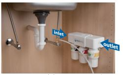
Onnect supply lines: insert tubing from the tee fitting into the inlet side and insert tubing from the faucet into the outlet side. Use diagram on the right to mark tubing depth to ensure they get inserted completely.
