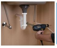
7 Use a 7/32" drill bit to drill holes for the plastic anchors provided. Carefully tap the anchors into the drilled hole with a hammer. Mount unit to the wall with the screws.
