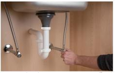
Unpack and unwrap contents. Turn off and disconnect the cold water supply.
