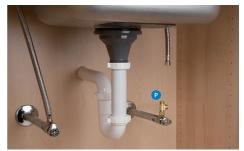
2 Attach threaded ends of supplied brass tee to the cold water supply line and shut-off valve; tighten using an adjustable wrench.
