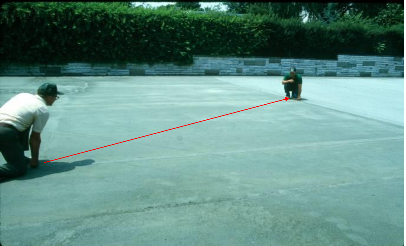
Checking Planarity
