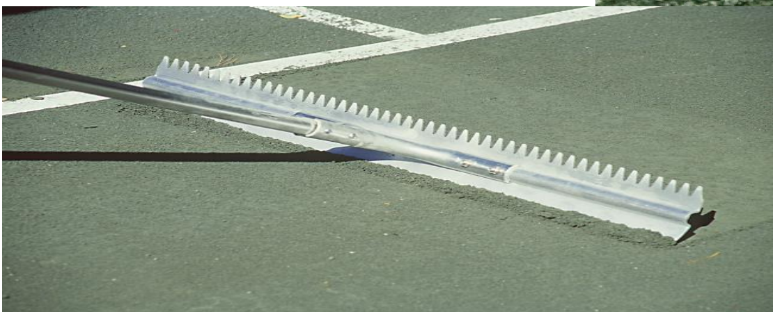
STEP 2 Repair divots & low spots
