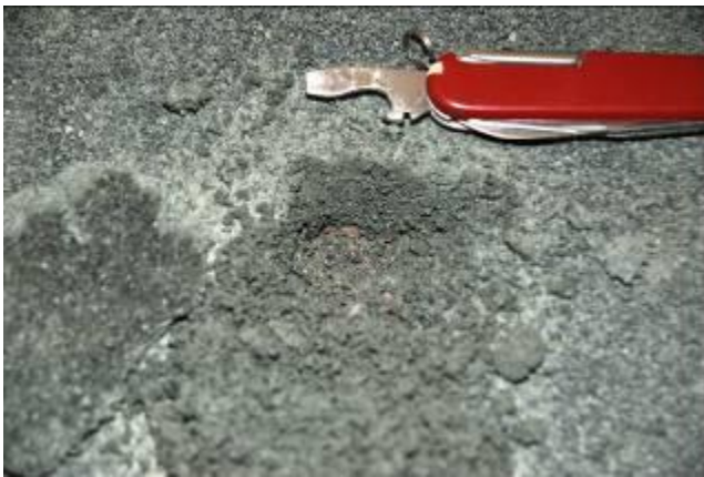
Photo 3: Good Surface Below Compaction
