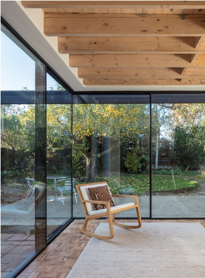
Existing Joists revealed
